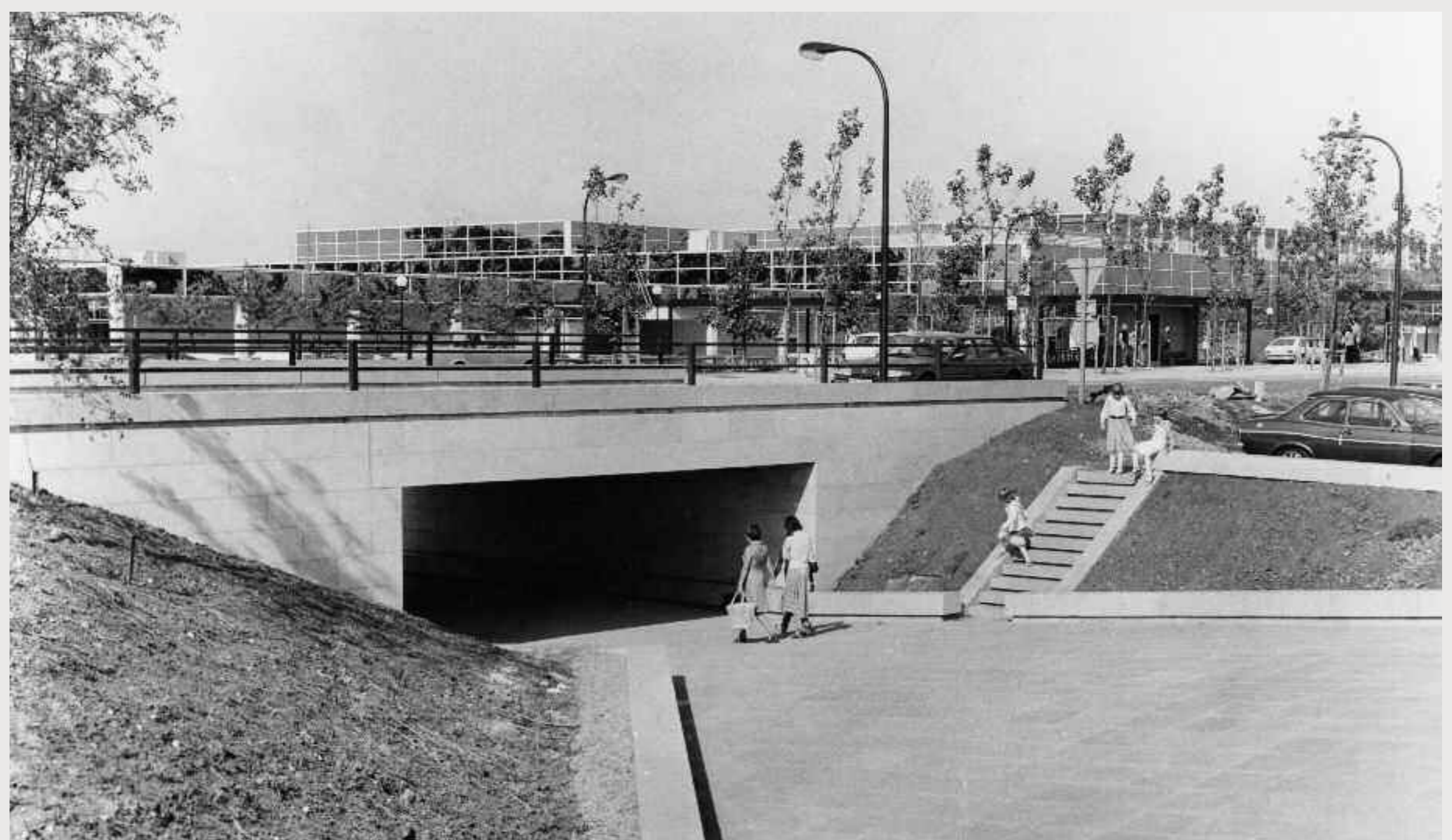
Underpass on Saxon Gate showing the Shopping Centre in background. Photograph by Ivor Leonard. Image copyright Homes & Communities Agency, courtesy of Milton Keynes City Discovery Centre.
