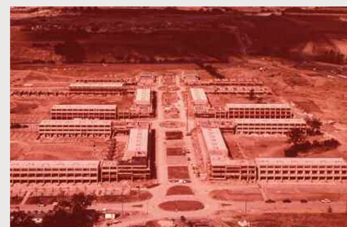
Fishermead housing development looking south, 1975. Image copyright of Homes & Communities Agency, courtesy of Milton Keynes City Discovery Centre.
