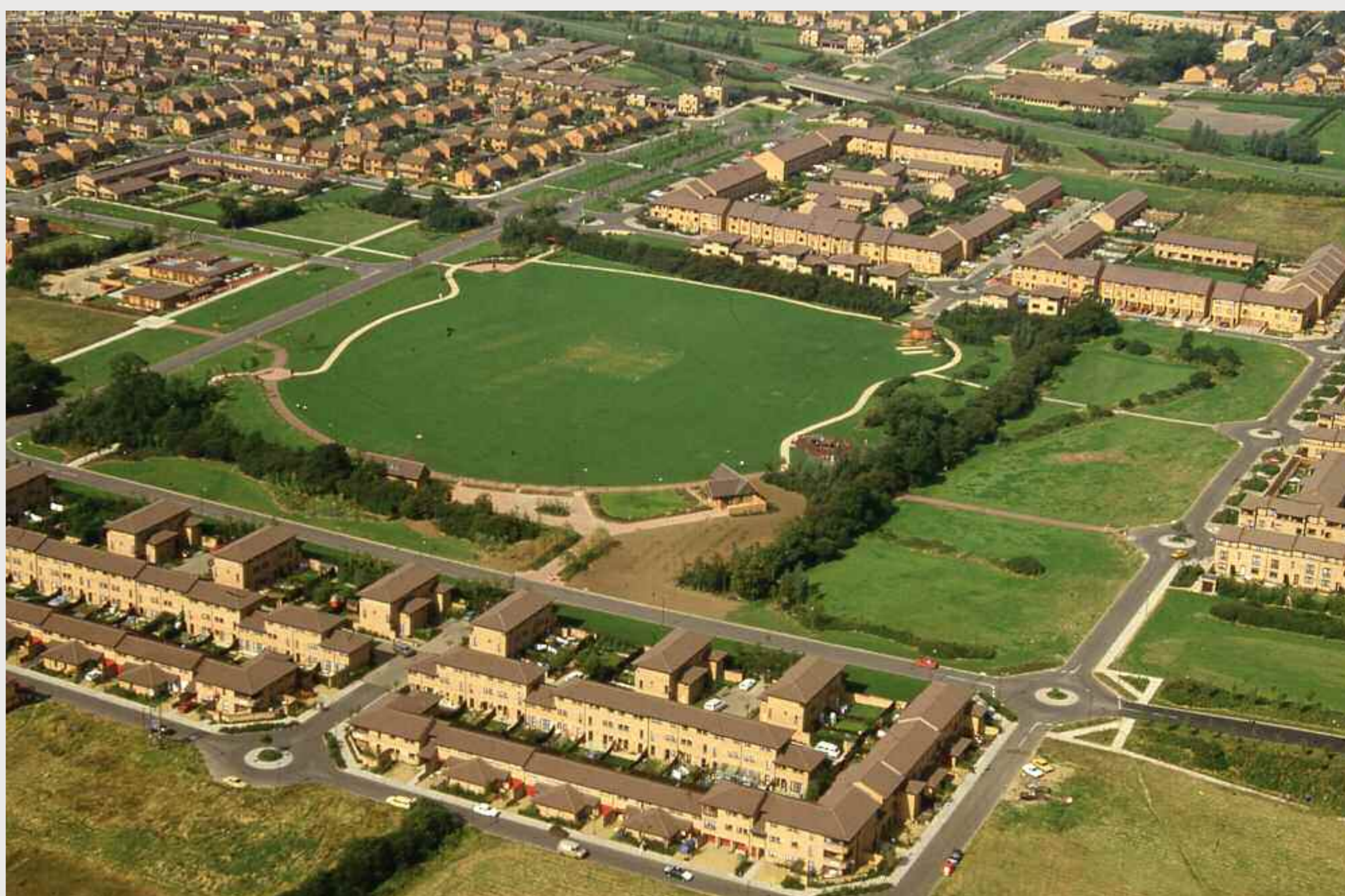
View of cricket pitch with housing and Cricketers pub. Image copyright of Homes & Communities Agency, courtesy of Milton Keynes City Discovery Centre.
