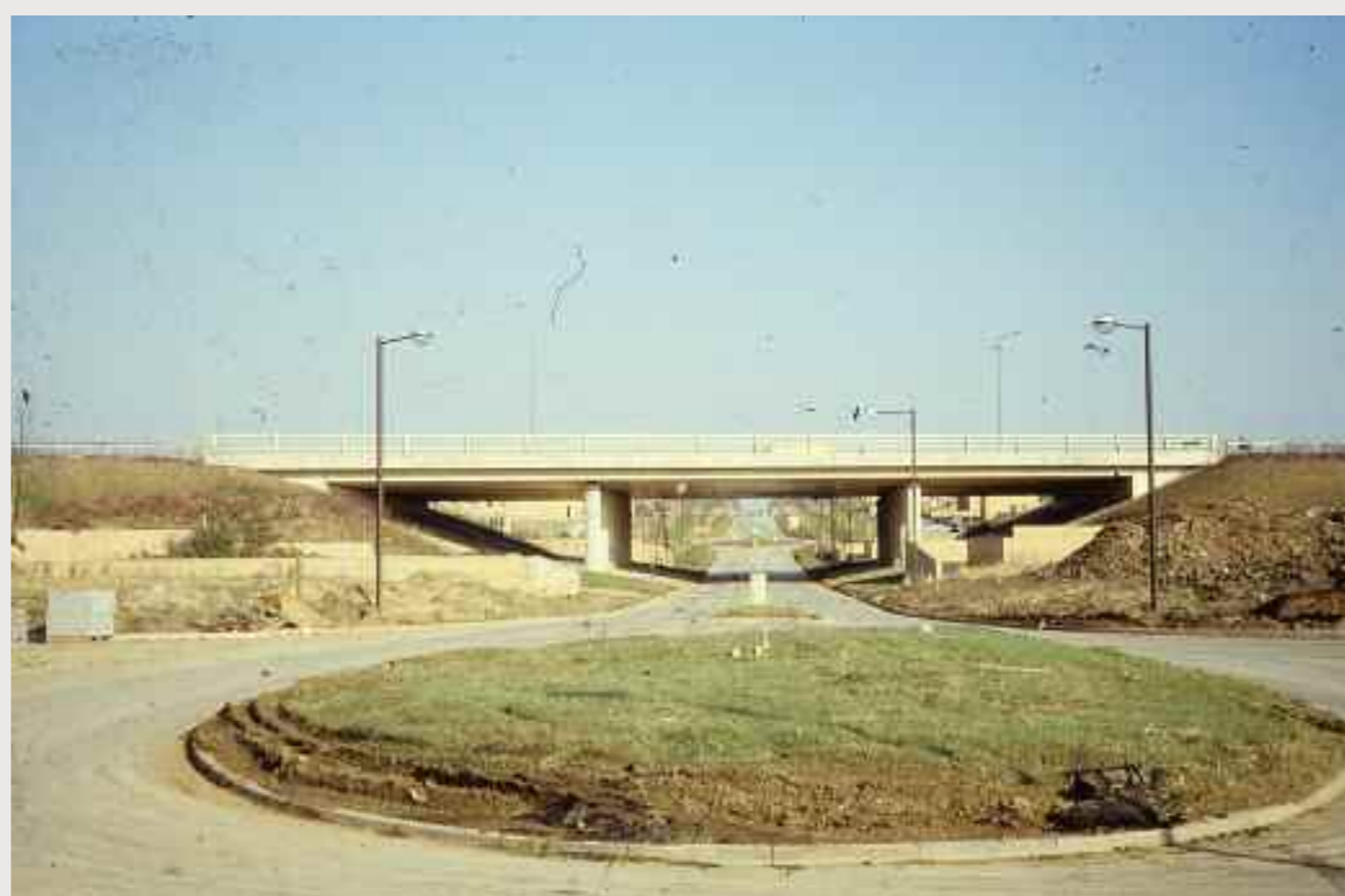
Under bridge below the V7 at Oldbrook and Fishermead. Image courtesy of Milton Keynes City Discovery Centre.
